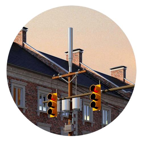
Today, small cells are being deployed that enhance existing cell towers by densifying wireless networks. This deployment provides the additional capacity and reduces congestion to accommodate the growing demand for mobile data.
